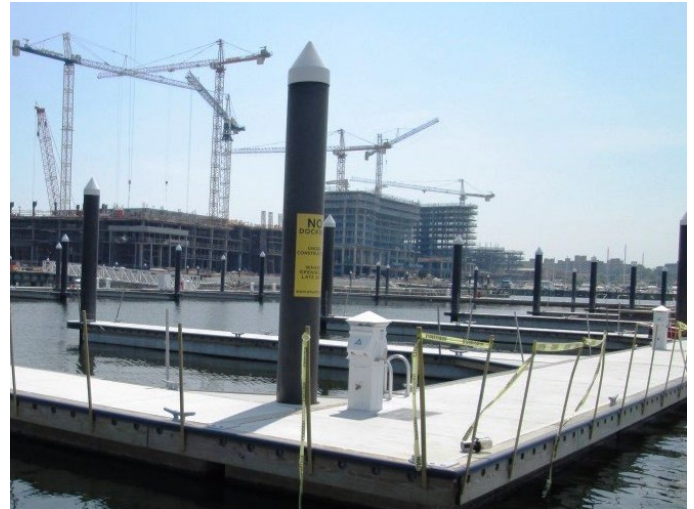
Boating Infrastructure Grant dock project, Wharf Marina, Washington, D.C.
